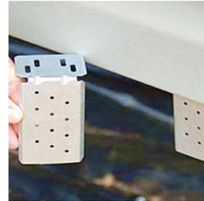
A wooden batten can be used, slightly off set from the edge underneath so the Top Trim Back is flush with the side of the home. **Do not screw directly to side of home.** Alternatively, we offer galvanised skirting brackets on our website.
