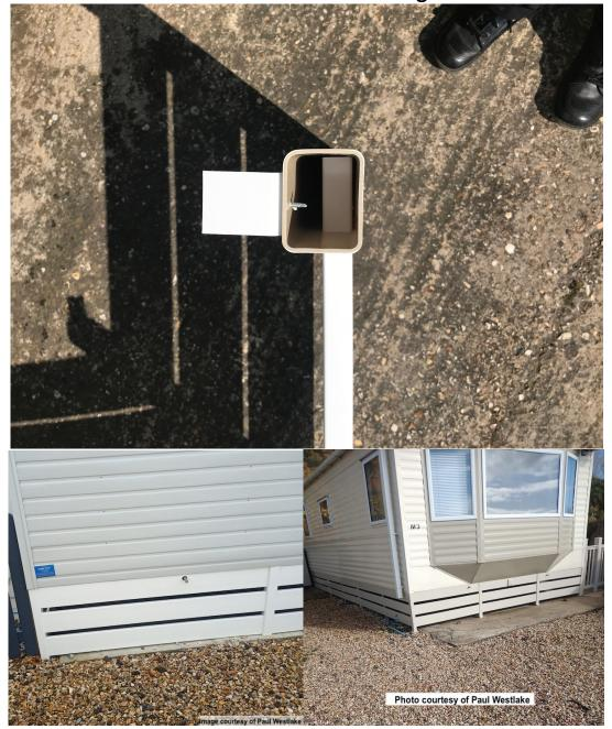
We the suggest temporarily fitting the opposite corner post in the same way and then stringing a line between the 2 to keep all the mid posts inline which should be fixed at equally spaced intervals between the corner posts at a maximum of 2410mm centre to centre of post. You can then work your way around the home adding the posts and fascia boards which are slotted into the prerouted ranch posts
