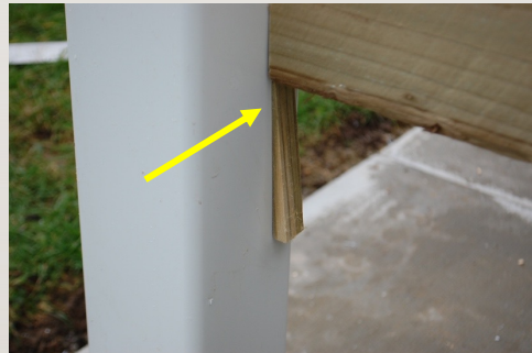
Use wooden wedge to make level if required
