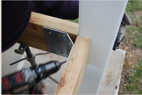
Pilot drill using a 6.5mm bit
