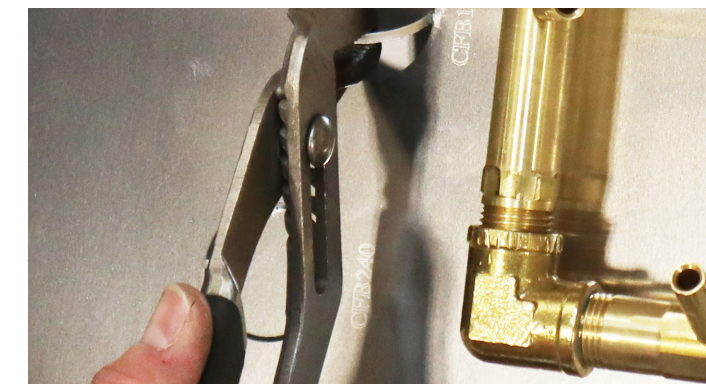
Photo 2: Breaking the Knockouts
