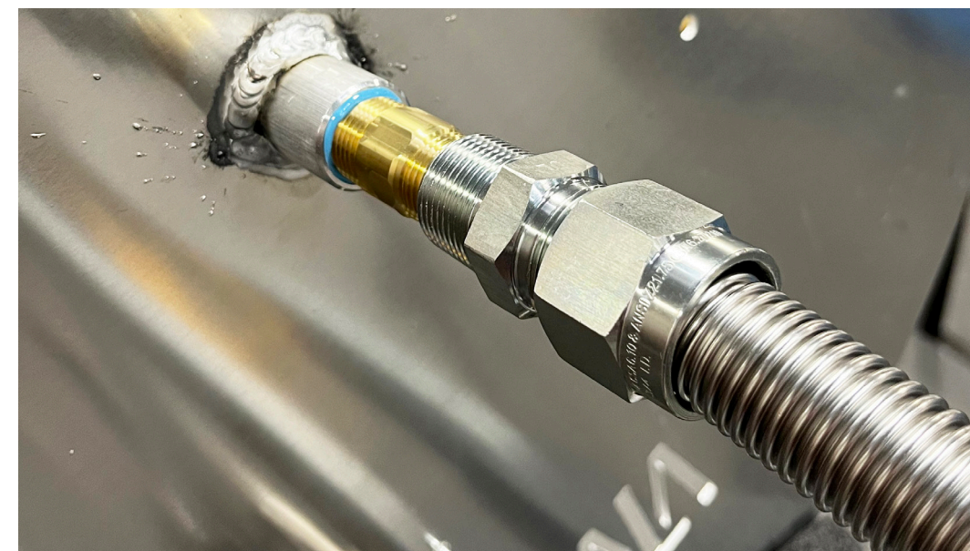
Photo 18: Connecting the Flex Line
