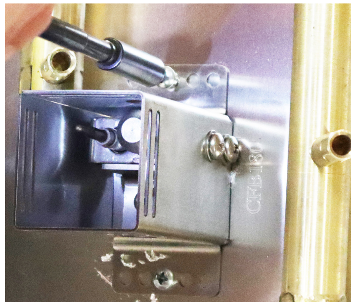
Photo 5: Securing the Pilot to the Plate/Pan
