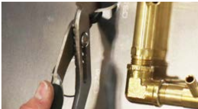
Photo 2: Breaking the Knockouts
