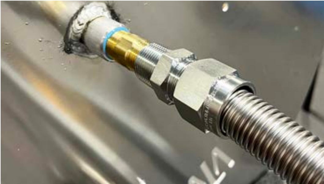
Photo 18: Connecting the Flex Line
