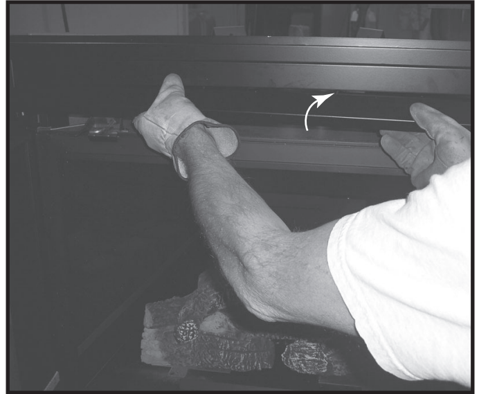
Figure 3. Install Hood
