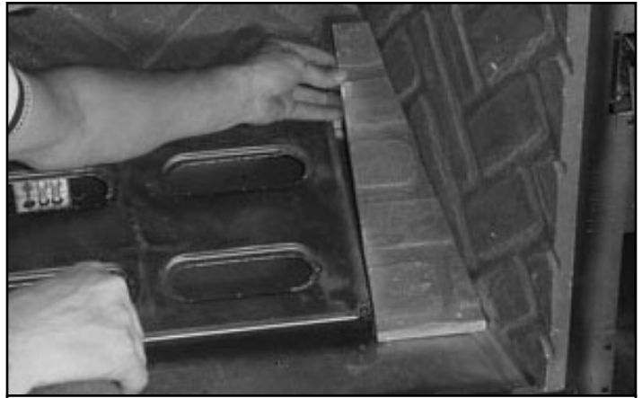
Figure 2.10 Removing Side Hearth Refractory
