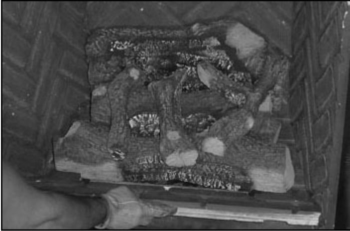
Figure 2.7 Removing Front Hearth Refractory
