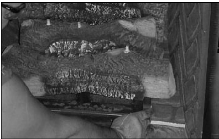
Figure 2.9 Removing Logs and Grate Assembly
