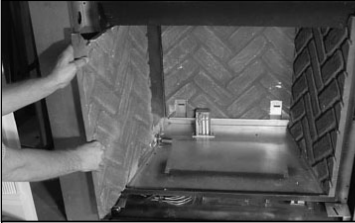
Figure 2.13 Removing Left Side Refractory
