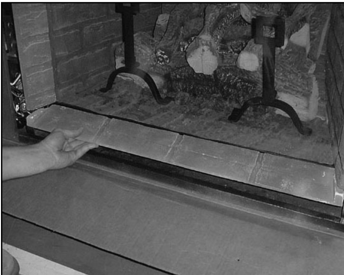
Figure 2.2 Remove Bottom Front Hearth Refractory
