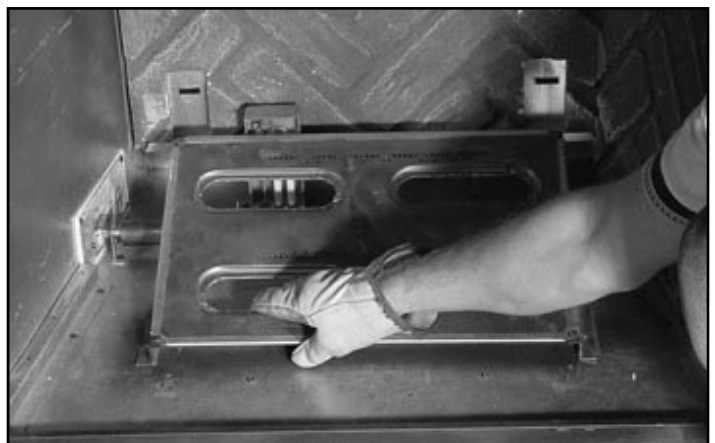
Figure 2.12 Sliding the Burner
