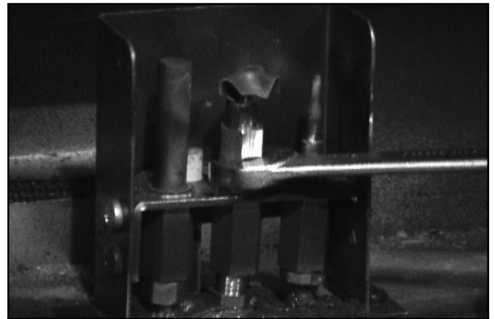
Figure 1.12 Loosen the Pilot Hood (CD & Designer Series)
