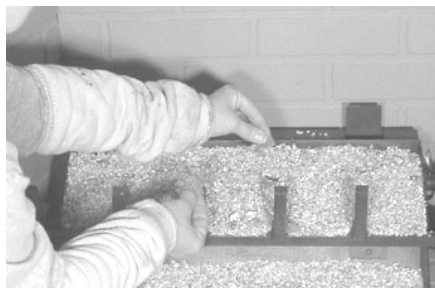
Figure 4c-Placing remaining rock wool
