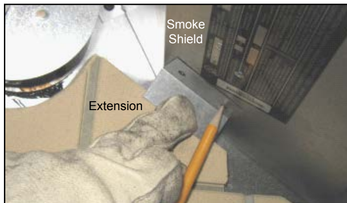
Figure 7 Place Retainer and Mark Holes
