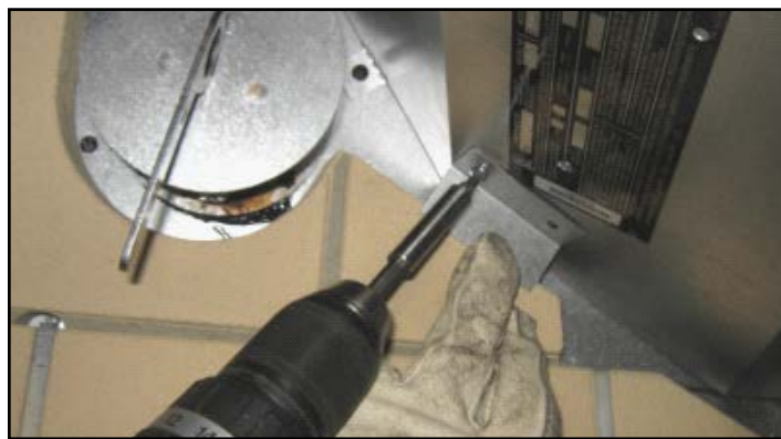
Figure 8 Attach Retainer
