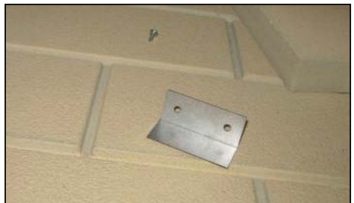
Figure 2 Stone Retainer and Screw
