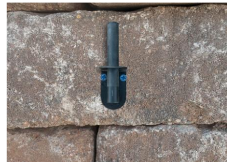
Figure 6.9 – Fasten down the bracket
