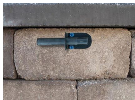
Figure 6.5 – Fasten down the bracket
