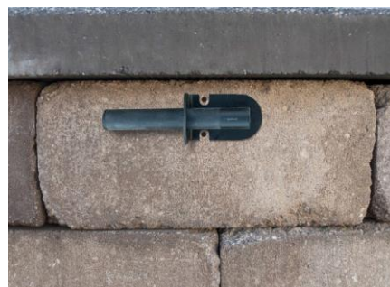
Figure 6.4 – Dry fit the bracket
