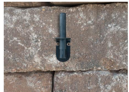
Figure 6.8 – Dry fit the bracket
