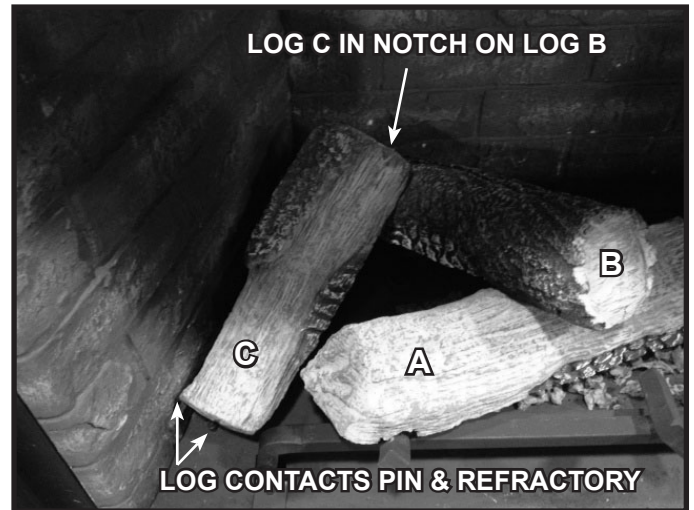
Figure 7. Log C Installed
