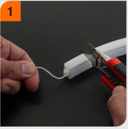
Use a sharp knife to cut the neon channel to the desired size. Before cutting, securely hold the string, then proceed to cut the channel slowly.
