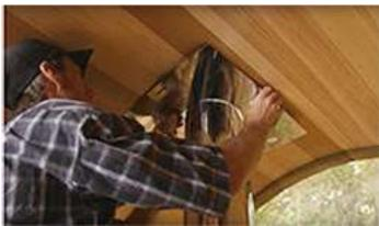
Get a helper to hold the chimney centered in the hole while you place the 2 flange pieces around the pipe.
