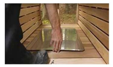
Install the floor plate centered between the benches at least 16" (41cm) from the inside groove of the dome.
