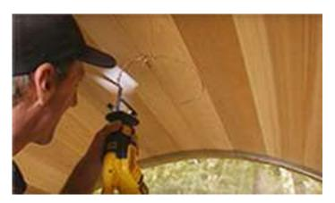
Start a hole inside your circle with a drill bit or other method, then use a reciprocating saw to cut out the circle as neat as possible.
