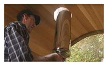
Slip the larger stove pie through the hole in the roof and then connect it to the extension pipe out of the stove.
