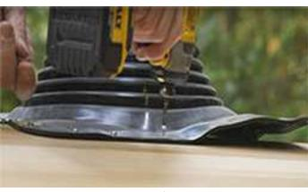
Using the provided 1" (25mm) stainless steel screws, secure the rubber flange to the sauna roof spacing the screws out as evenly as possible.
