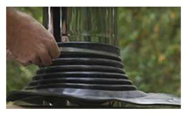
Place the tightening clamp around the rubber flange and tighten up with screwdriver.
