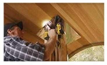
With the pipe centered, secure the flange pieces to the roof with the provided 1" (25mm) screws in the 2 slotted grooves.
