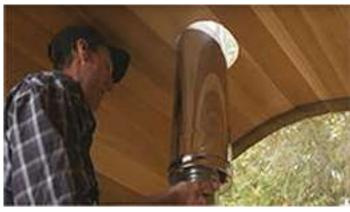
Place a piece of the pipe through the hole to make sure it fits before moving on to the next steps.
