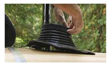
Pull the rubber flange over the seam where the 2 pipes connect.
