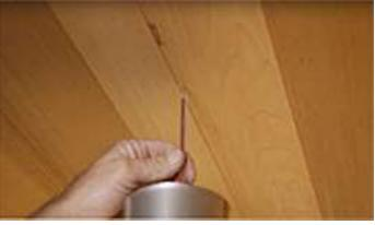
Once the extensions are connected close to the roof of the sauna, locate the center of the pipe and use a pen or pencil to mark the roof.
