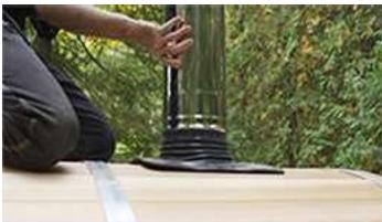
Slide the top chimney piece over the bottom chimney pipe.
