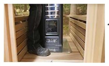
Using 2 people, place the Harvia M3 Heater centered between the benches on the floor plate.
