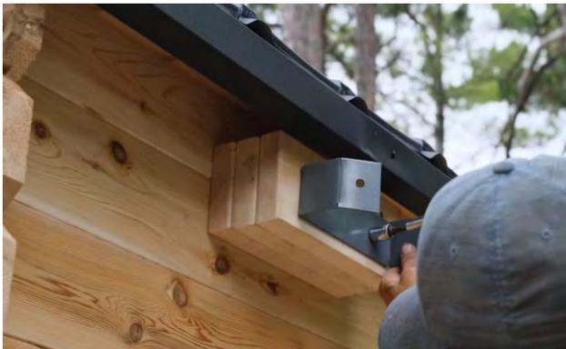
Mark the center of the 3<sup>rd</sup> support piece and install the chimney support bracket centered on this mark with the included lag screws.
