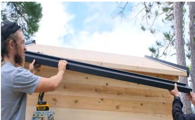
Place the long metal trim pieces on the sides of the roof and secure with the included short black screws.
