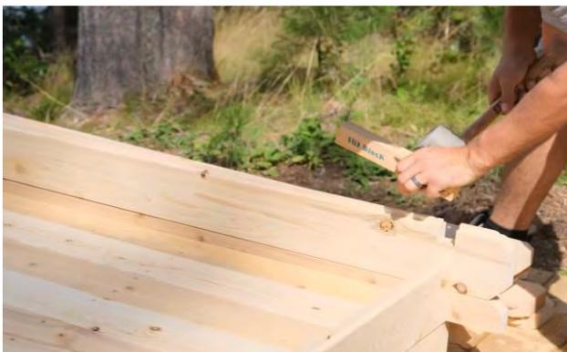
Now place a full-length stave at the rear of the sauna and tap the tongue and groove together to make sure it is tight and secure with a 5" (127mm) screw into the notch at either end.
