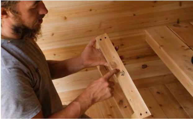
Place the small bench support on the other end, make sure the side labelled “top” is upward.
