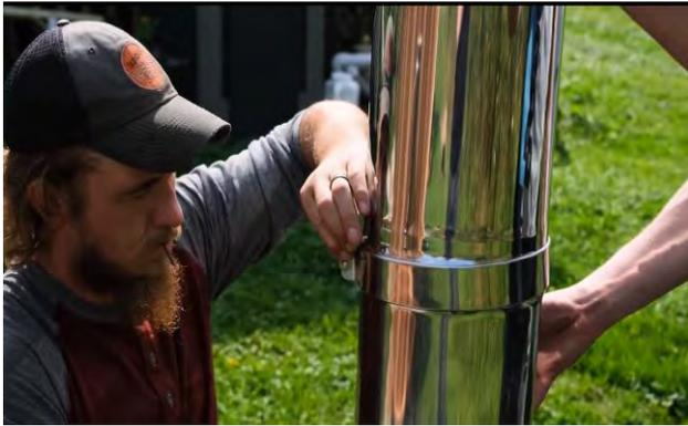
Attach the support strap around the 2 chimney pipes and tighten up.
