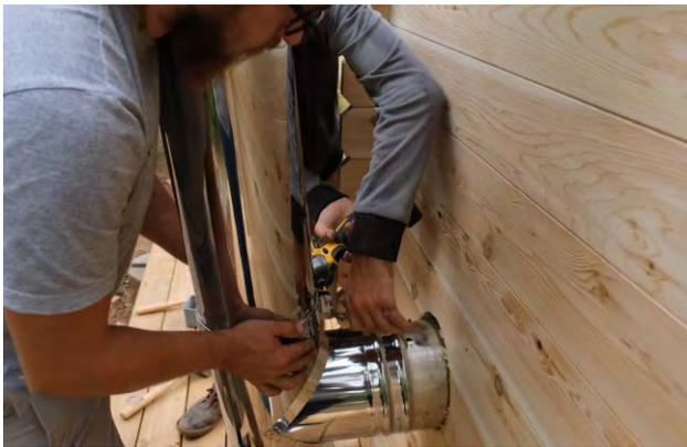
Attached assemble chimney pieces to the "T" coming out the back of the sauna and secure with a support band.
