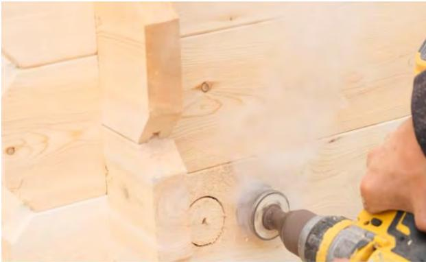
Mark the vent inlet hole positions on the side wall of the sauna, next to the stove, and drill out with a 2" (51mm) hole saw.
