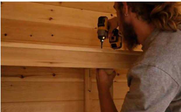
Align the bench supports to the slats on bottom of bench.
