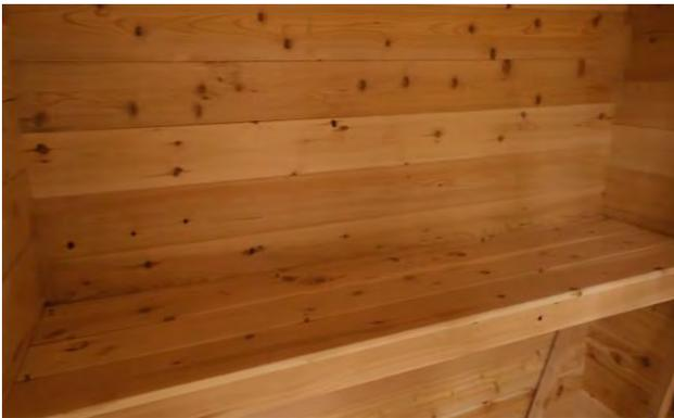
Place the top bench onto the supports and secure with 2 ½" (64mm) screws into the wall mount bench brackets.
