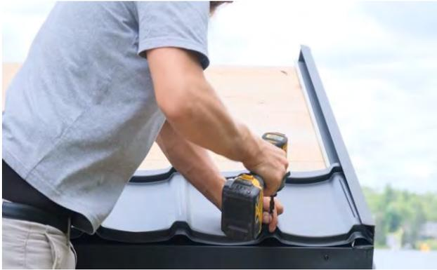
Start applying the metal shingles by sliding the shingle under the side metal trim piece and flush with the edge of the side trim and then secure using the included roofing screws.
