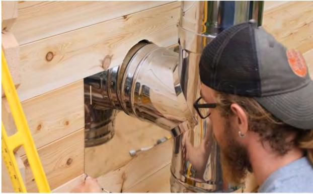
Install the bottom half of the exterior chimney shield with the provided screws.
