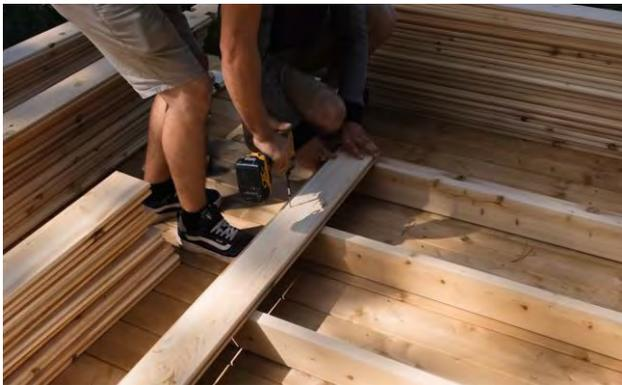
Secure with 2 - 3" (76mm) screws per support.
