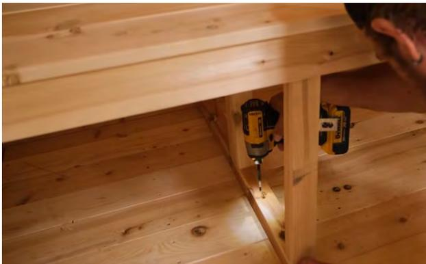
Screw the bench supports to the floor and back wall using 2 ½" (64mm) screws.
