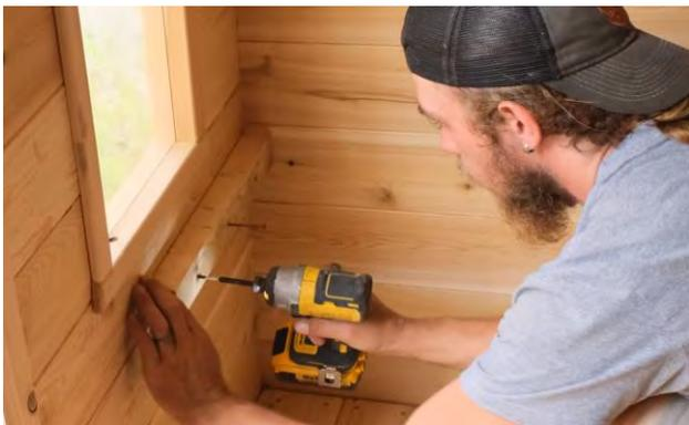
Mount the remaining wall mount bench bracket flush to the line of the bench and secure with 3 - 2 ½" (64mm) screws.
