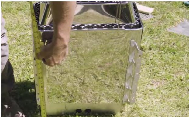
Measure the height of the mounting holes and add 6". (152mm)
