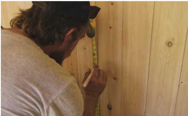
Transfer the measurements to the back wall of sauna.
