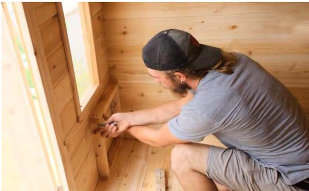
Place the small bench support against the wall and mark the top and the front as in previous steps.
