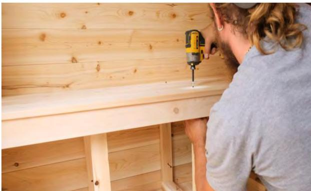
Line up the supports and secure the bench to the supports and the supports to the floor and side wall in the same manner as previous steps using 2 ½” (64mm) screws.
