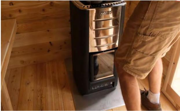
Place the stove onto the heat shield.
