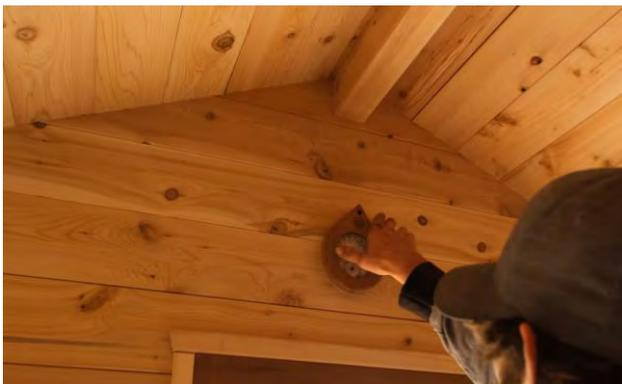
Install the optional Thermometer using a 1 ½" (38mm) screws.
