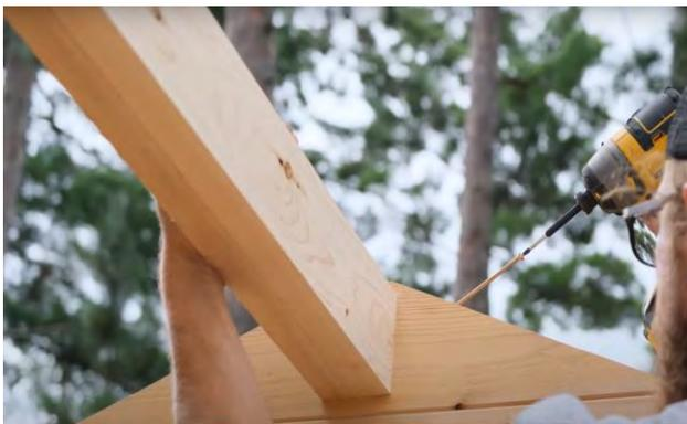
Secure each end with a 5" (127mm) screw on each side of each triangle piece.
