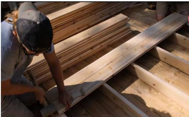
Align the next floor stave up to the edge of the first one and tap the tongue into the groove.
