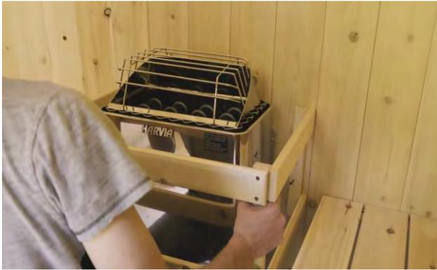
Center the guard around the heater and secure to wall with the pre placed screws.
