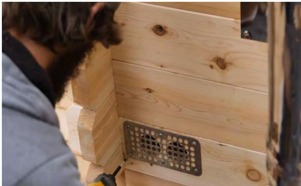
Using 1 ½" (38mm) screws, screw on the vent cover.
