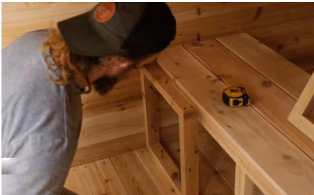
Screw the bench support to the benches and side wall using 2 ½” (64mm) screws.
