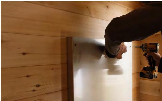
Secure the heat shield to the wall with 6 - 1" (25mm) screws.
