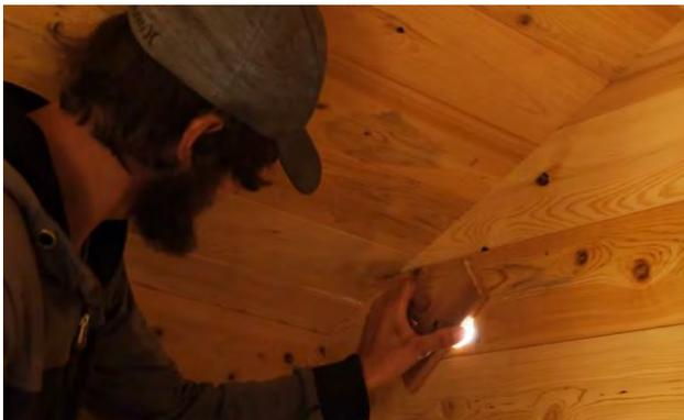
Use a 1 ½" (38mm) screw and attach the vent board on the inside of the sauna making sure it is tight but can still be turned.
