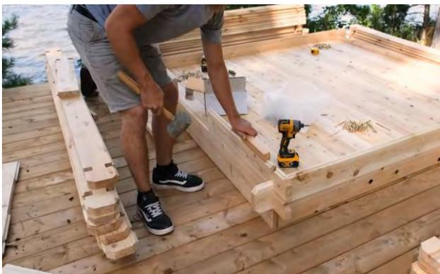
Place one of the medium length wall staves at the front of the sauna and using the provided "hit block" tap it so the groove goes tight into the tongue of the front starter stave.
