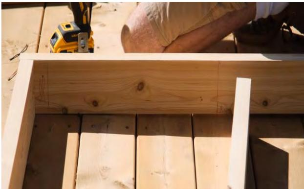
The front and back pieces will be “marked” where each of the base supports will be placed.
