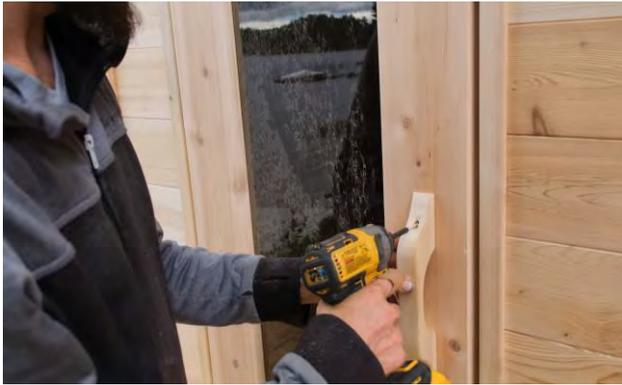
Install the outer door handle (small) at the desired height using 2 - 2 ½" (64mm) screws in the pre-drilled holes.
