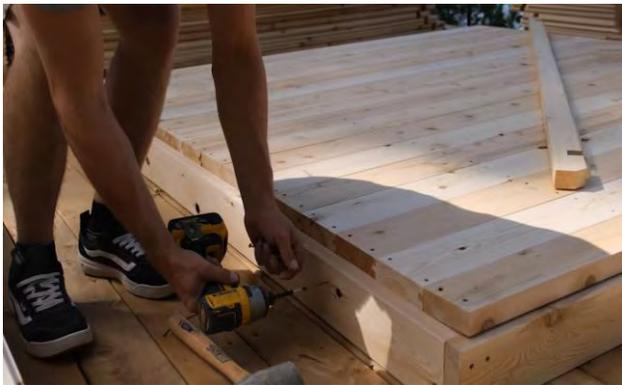
Place 3 -3" (76mm) screws into each of the side supports.
