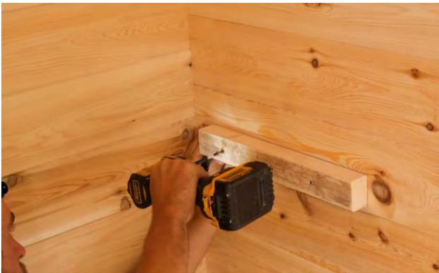
Mount one of the wall mount bench brackets flush to the line on the upper bench and secure with 3 – 2 ½" (64mm) screws.
