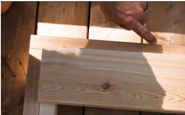
Ensure the "floor Starter" stave is flush with the inside of the front and side base plates.
