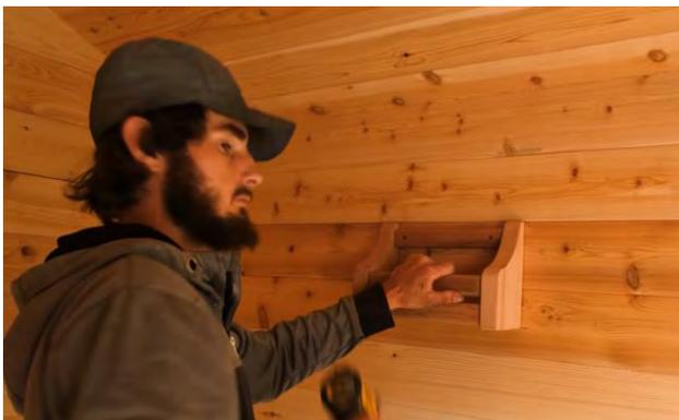
Install the optional shelf at the desired location and secure with 2 - 1 ½" (38mm) screws.
