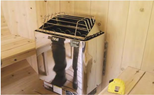
Hang the heater on the 2 screws and tighten to secure stove in position.
