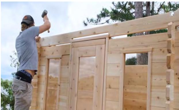
Secure the other full length front wall stave labelled "Door" above the windows and door and secure with 5" (127mm) screws into the notches in the same manner as the previous steps.
