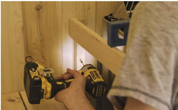
Ensure the guard is level and secure the other side.
