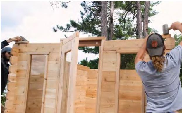
Place a medium length front wall stave above each window and secure using a 5" (127mm) screw into each notch.
