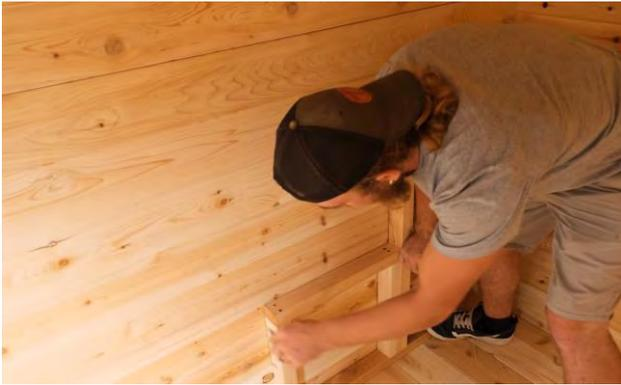
Start the assembly of your benches by placing the 2-tier bench support along the wall.
