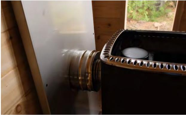
Place the chimney through the hole, then through the heat shield (hole towards the bottom), then into the stove.
