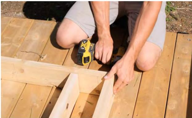
Insert 2 – 3” (76mm) screws into the end of each base stave.
