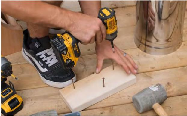
Place 3 – 3" (76mm) screws into each of the 3 chimney support boards.
