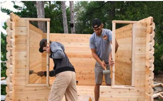
Place your windows onto the front wall and ensure the staves are fully inserted into the grooves.
