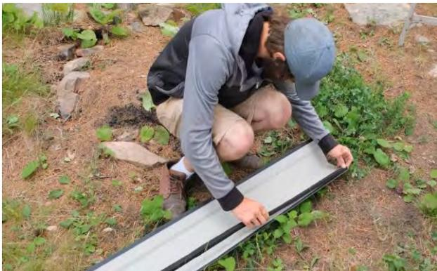
Reveal the adhesive side of the M-seal and apply it to the inside edges of the roof ridge cap.
