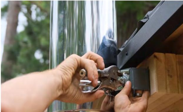
Push the chimney in until it aligns with the top support bracket and secure it with a support band and the included bolt and washers.
