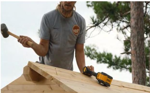
When you reach the top of one side, use the wide stave without the groove on the top.
