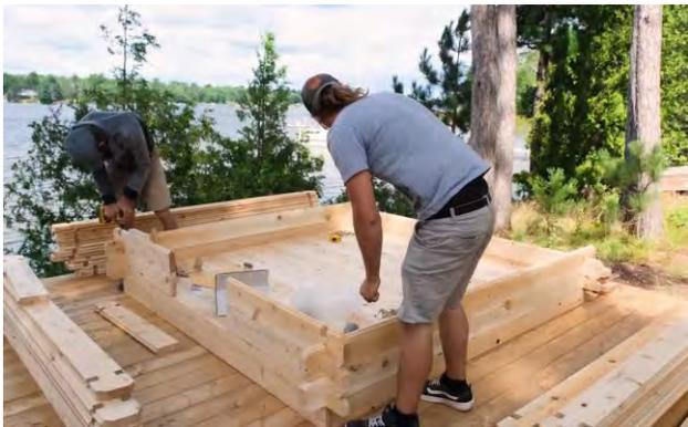
Continue with the front wall by placing one of the medium length wall staves on both ends and tapping them so the groove goes tight into the tongue of the front starter stave and secure it with a 5" (127mm) screw into the notch.
