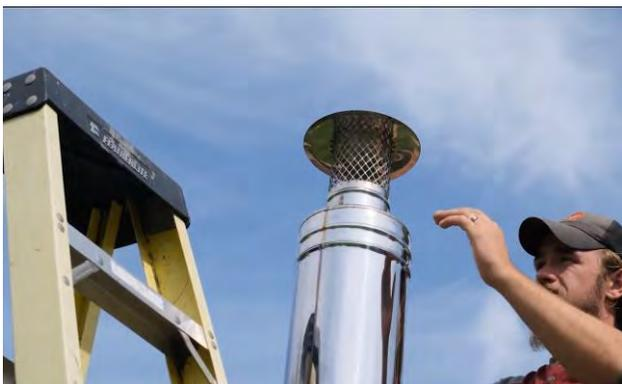
Install the cap on the top of the assembled chimney.
