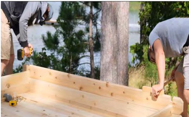
Continue this process using a full-length stave at the rear of the sauna and tap the tongue and groove together to make sure it is tight and secure with a 5" (127mm) screw into the notch at either end.
