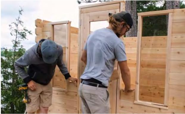
Slide all the small front wall staves between the door and windows and ensure they are tight to each other by tapping with a mallet.
