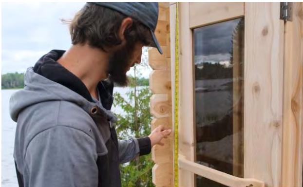
Install the inner door handle (large) horizontally at the desired height. Ensure the handle is level and secure using 2 - 2 ½" (64mm) screws in the pre-drilled holes.
