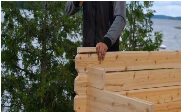
Repeat the process of placing and securing the sides, back wall staves and short front wall staves until the short staves are 8 staves high.
