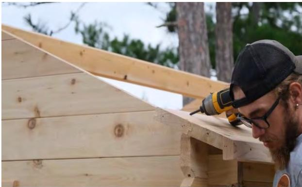
Align the notch with the edge of the triangle pieces and use 2 - 3" (64mm) screws on each end and 5 - 3" screws from the roof board into the side wall.
