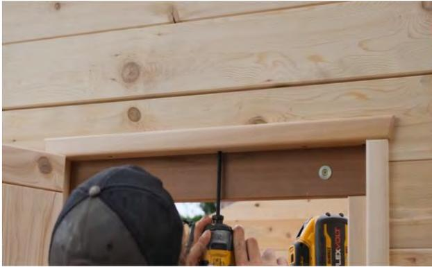
Use a 5" (127mm) screw in between the previously placed screws in the top of the door frame to pull in the middle of the triangle piece.
