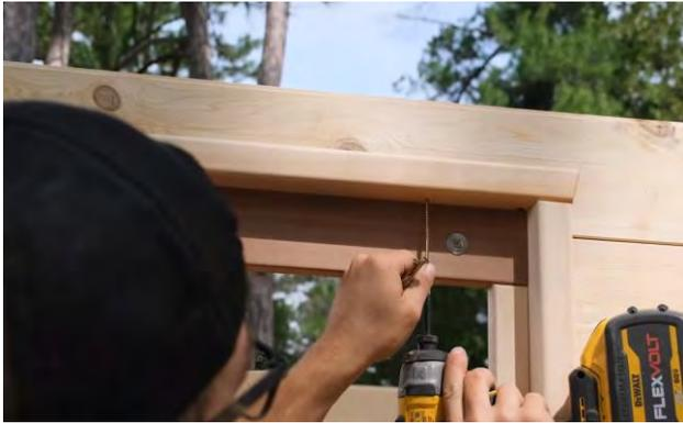
Insert 2 – 3" (64mm) screws into the top of the door frame as shown.
