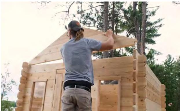
Place the front and rear triangle front pieces onto the sauna.
