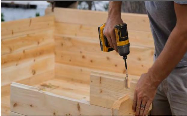
Place a short front wall stave on either side of the front wall and secure with a 5" (127mm) screw in each of the notches.
