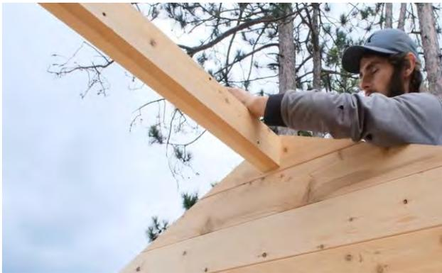
Place the center roof support beam into the slots on the top of the triangle pieces.
