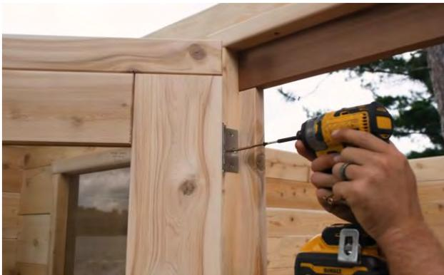
Place a 3" (64mm) screw through the middle hole on the 2 hinges and then centered in the frame between the 2 hinges.
