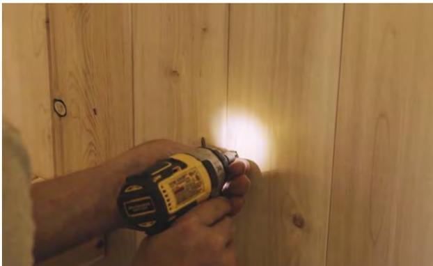
Install the two  $\frac{1}{4}$ " x  $1\frac{1}{2}$ " (6mm x 38mm) hex head lag screws (supplied with the heater) into the holes.
