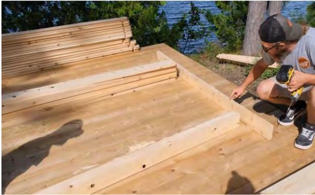
Start the assembly of your Georgian Cabin by laying out the front and back base plates and the 8 – base supports.
