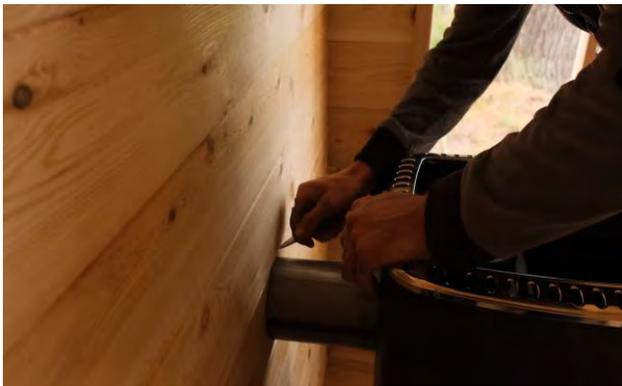
Place the short metal pipe into the back of the stove and mark it where it meets the wall.
