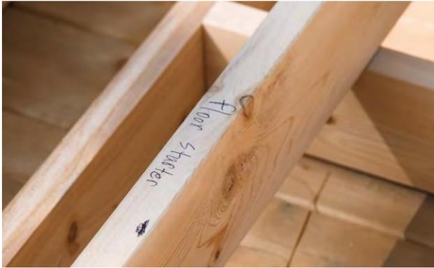
To start the assembly of the floor, locate the stave that is labelled "Floor Starter"
