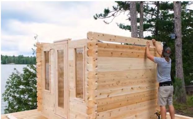
Insert a rear wall stave and a side stave on either side of the sauna and secure using 5" (127mm) screws into the notches on each end of the staves.
