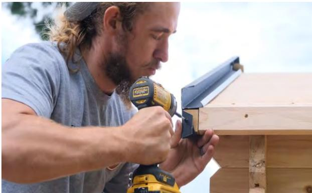
Fold over the ends of the metal trim pieces and secure with the included black short screws.
