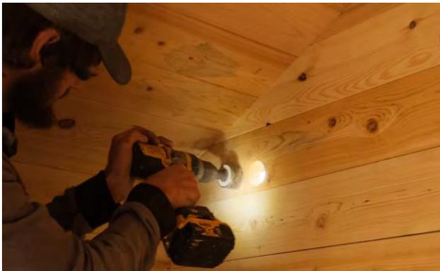
Mark the vent outlet hole position high up on the back wall.
