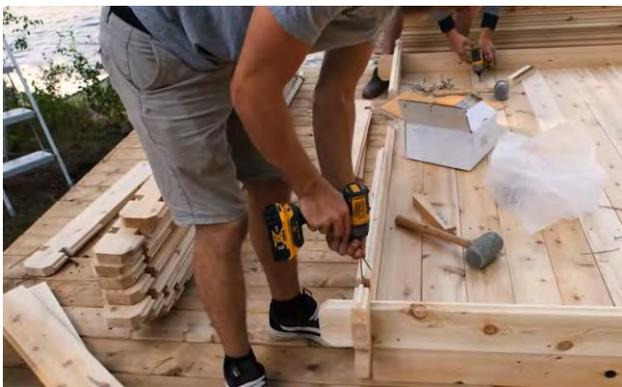
Insert a 5" (127mm) screw into the notch to secure it to the starter stave below.
