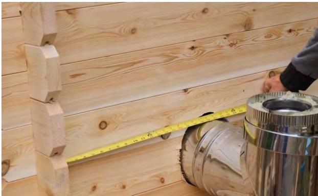
Measure the distance from the wall to the center of the chimney.
