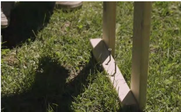
Place 2- 2 ½" (64mm) screws into the pre-drilled holes on either side of heater guard to prepare for mounting.
