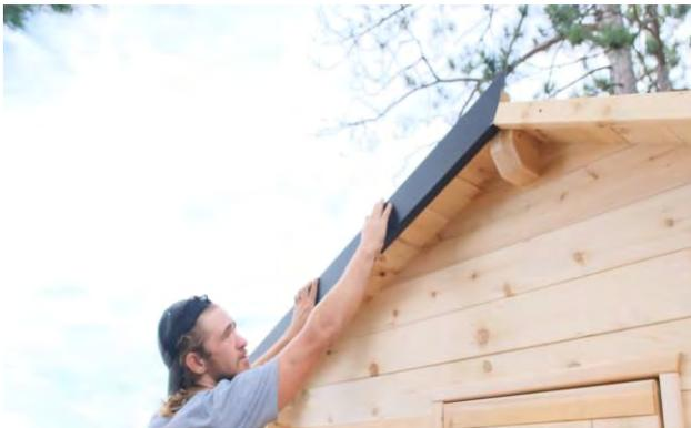
Secure the front metal trim pieces onto the wood trim pieces and secure on the face and underneath with the included short black screws.
