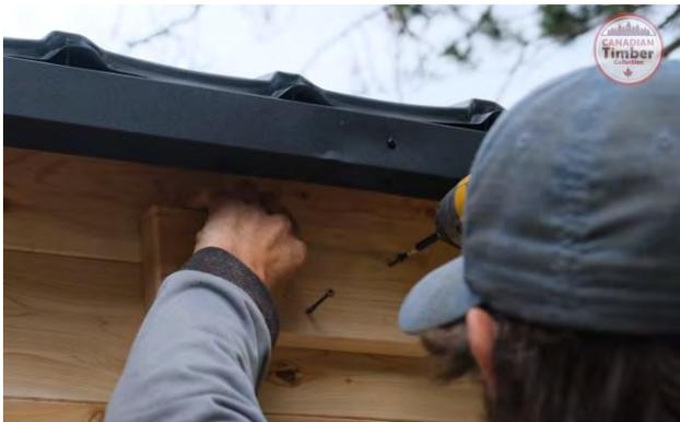
Secure the support to the wall lining up the center to the mark placed on the wall.
