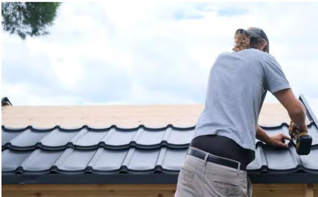
Continue adding the shingles up the roof overlapping the previous row securing with roofing screws on every ridge until you get to the last row needed.
