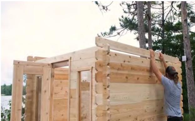
Place the side wall stave with the tapered edge on the side wall and secure in the notches with a 5" (127mm) screw on both sides of the sauna.
