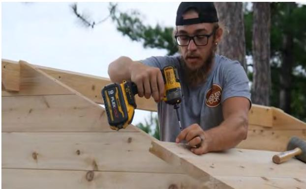
Start placing the roof staves going up the roof and tap into each other, secure with 2 - 3" (64mm) screws into each end.
