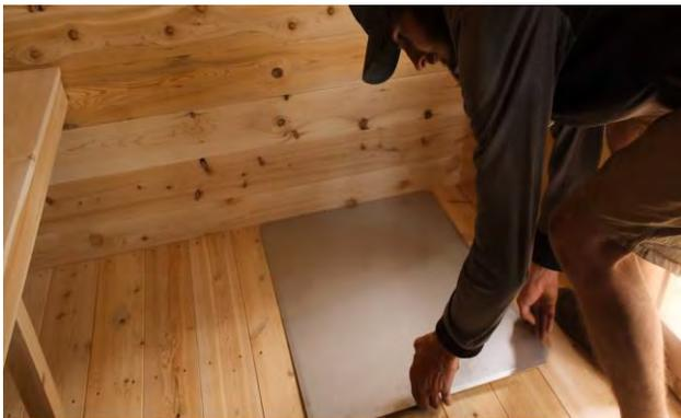
Place the heat shield on the floor where the stove will be.
