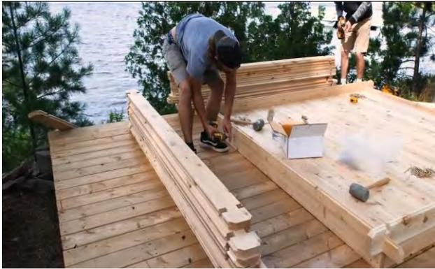
Fasten the front and rear starter staves with 2 - 3" (76mm) screws to secure it to the floor.
