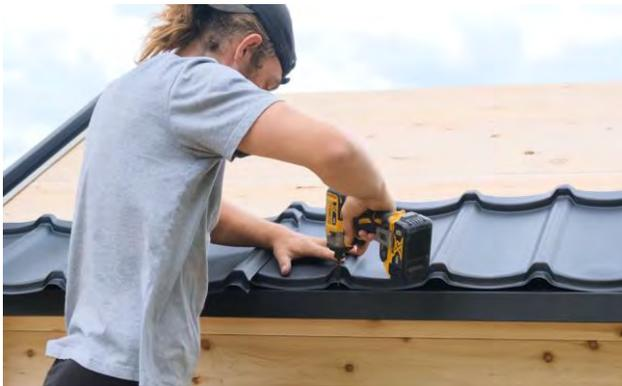
Overlap the panels one ridge and continue securing to the roof to the other side of the sauna.
