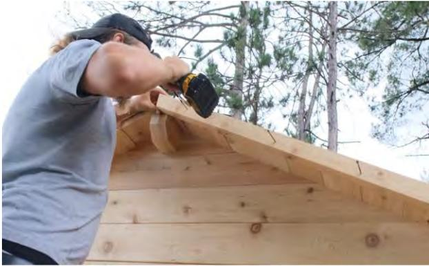
Pre-place 4 – 3" (64mm) screws into the front trim pieces and secure to the roof staves.
