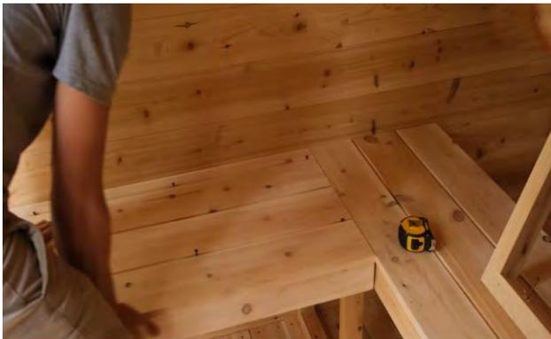
Place the bench on the supports and secure with 2 ½” (64mm) screws.
