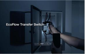
MANUAL MODE: In MANUAL MODE, after load shedding begins, switch manually to the backup power source through the full disconnect "off" position. Make sure you do not exceed the maximum operating power of the Portable Power Station. Manual mode is recommended for nobody at home or when you are sleeping at night.
