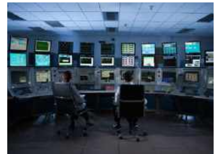
VIDEO SURVEILLANCE ROOM
