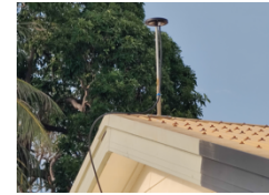
Example Roof Install of GNSS Antennae
