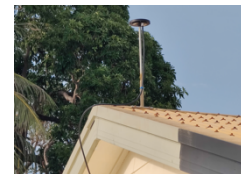
Example Roof Install of GNSS Antennae
