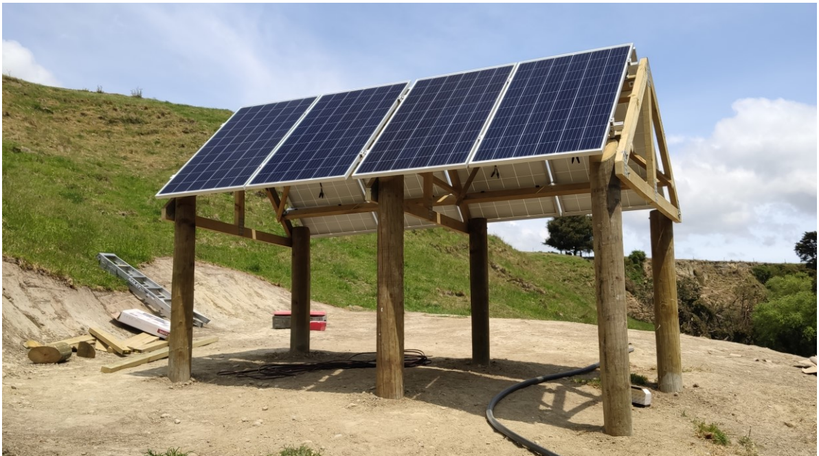
8 panel East/West twin React pump install
