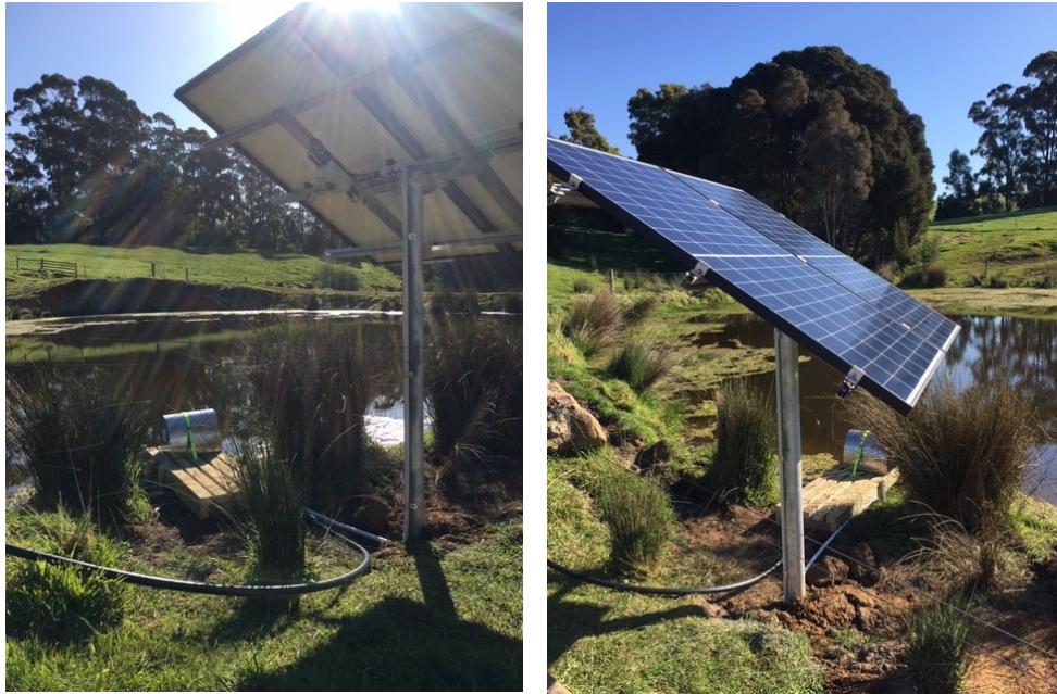
4 panel React pump ground mounted adjacent to a farm pond
