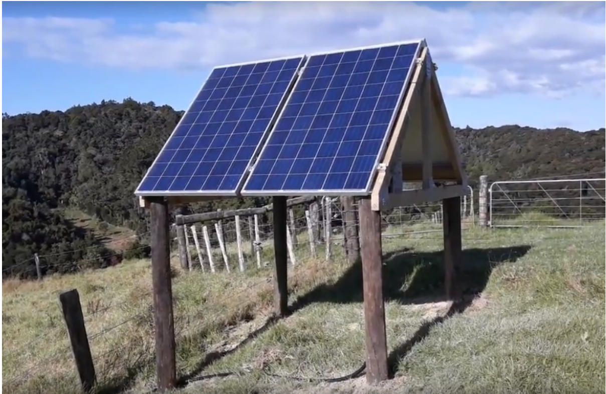
Typical East/West Truss mounted array remote from the React pump location
