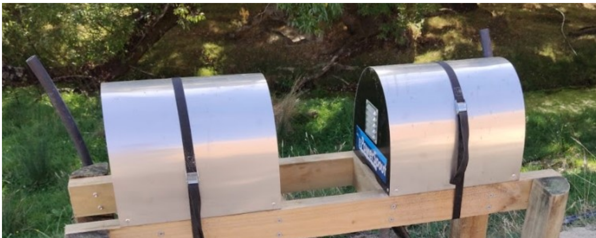
Note valve riser pipes for priming of each suction line
