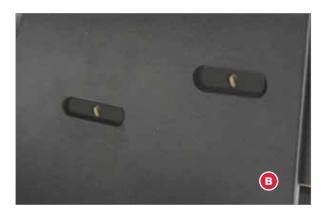
With the mounting holes aligned, insert a single M6 x 1.0 x 40 hex head bolt (K) through a M6 x 19 x 1 washer (J), then through one of the four exposed holes in the dust collection guard mounting bracket (B) and extension table, and then through a second M6 x 19 x 1 washer (J) and a M6 x 1.0 nut (L). Only finger-tighten the nut at this time.
