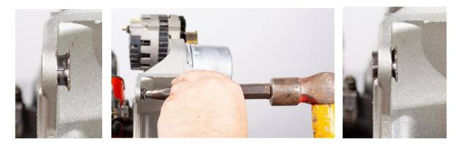
Step 4. With a hammer and punch drive the split sleeves back. This allows the compressor assembly to be installed and squared to the front of the bracket without interference.
