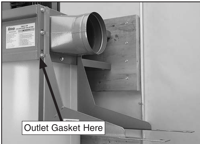
Figure 14. Outlet port and filter L-braces installed.
