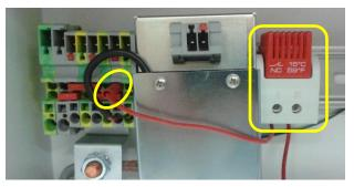
Install the Gray Power Connector and Green Ground Connector onto the DIN Rail next to the Thermostat. Ensure Power Connector (Gray) is to the left of the Ground Connector and next to the Thermostat.
