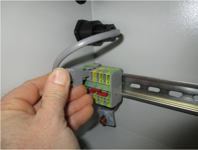
Figure 19: DC Cable to DIN rail
