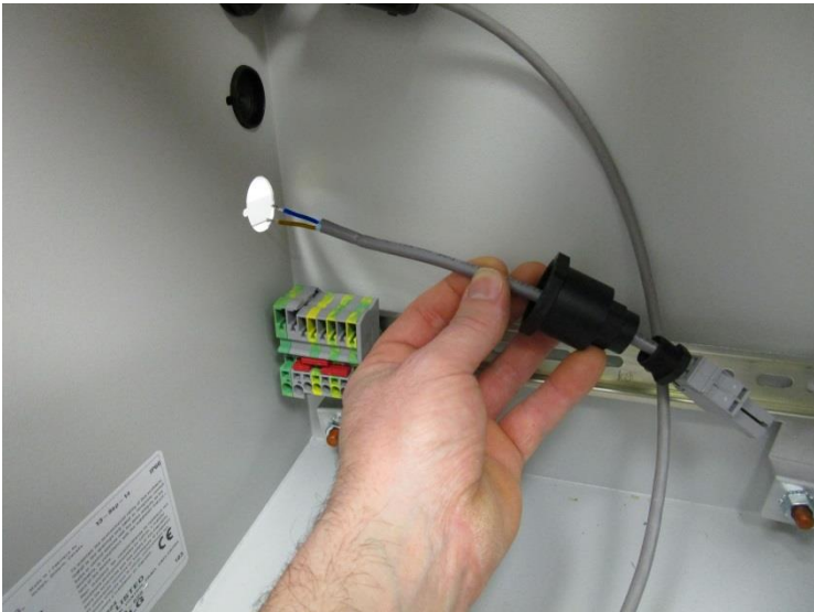
Figure 14: DC Cable Preparation
