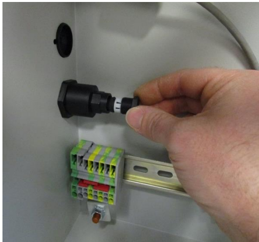
Figure 18: DC Cable Gland Nut
