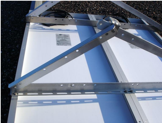
Figure 9: Assemble the Solar Cells on the Mounting Frame
