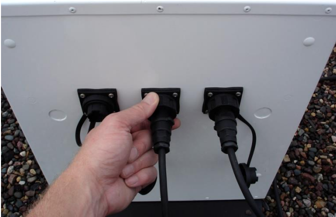
Figure 11: Connect Solar Cells to Battery Enclosure Box
