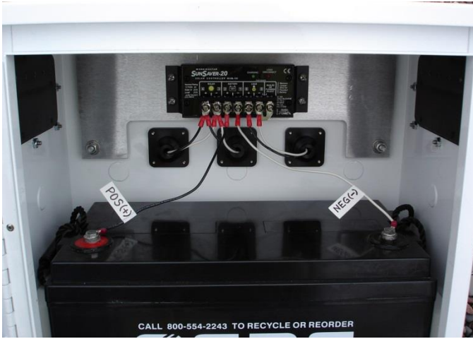
Figure 2: Install the Solar Battery and Connect to Controller
