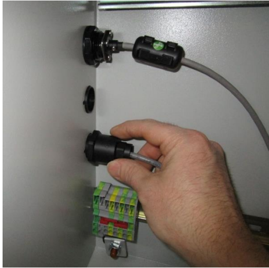
Figure 17: DC Cable Backshell
