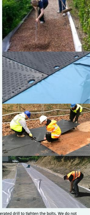
We recommend using either standard spanners, a wrench or a battery operated drill to tighten the bolts. We do not advise using air-drills as this can cause over over-tightening of the bolts. Please be sure not to over tighten bolts, as this can cause cross-threading and damage to the connectors. Additional reinforcement plates can be used for longer term or heavy weight projects.
