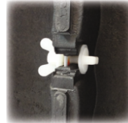
Single nylon fixing secures panel to base (view from underneath)
