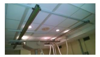
The next picture is from the same hospital. When this radiology room was remodeled, we again consulted our original drawings and calculations before mounting <u>P5500T rails</u> below the existing grid to support new GE equipment.
