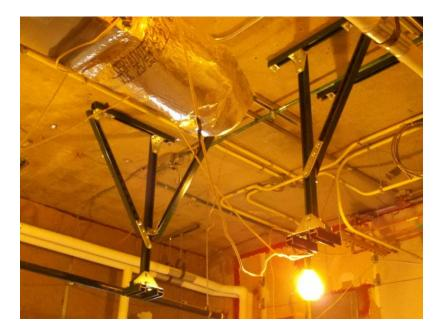
Surgical lighting systems are much larger (most are in the 24" diameter range), and of course, much heavier. Unistrut support structures surgical lights typically consist of four vertical members and up to eight braces as shown in the photo below:
