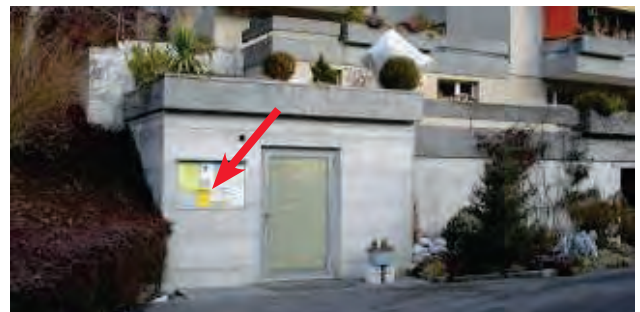
Bürgstrasse Nr. 23, an BKW Trafostation
