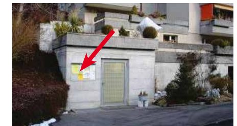
Bürgstrasse Nr. 23, an BKW Trafostation
