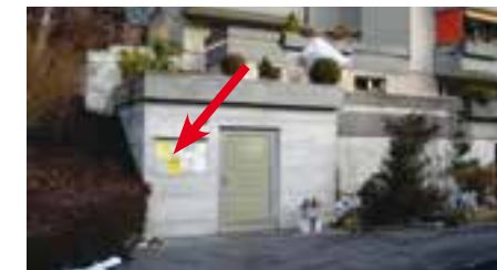
Bürgstrasse Nr. 23, an BKW Trafostation
