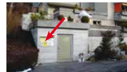
Bürgstrasse Nr. 23, an Trafostation
