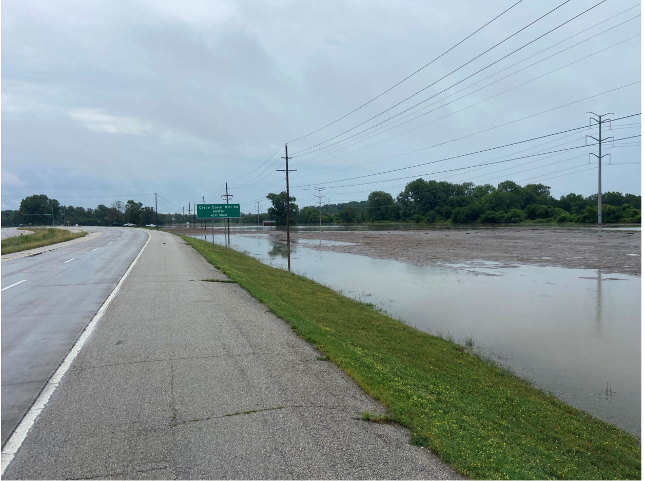
July 26, 2022, flooding of Creve Coeur Mill Rd.
