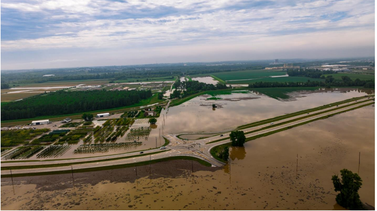
July 26, 2022, flooding at Marine and Hwy 141.
