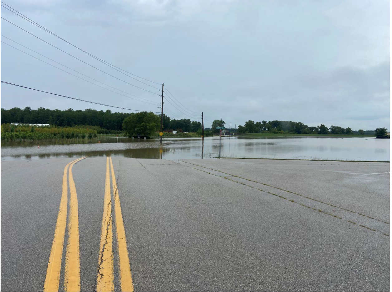
July 26, 2022, flooding of Frontage Rd.
