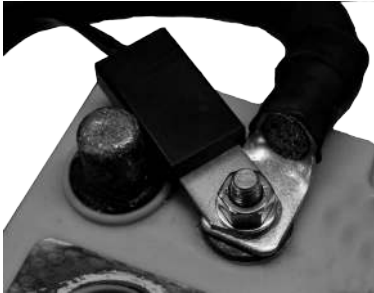
Fig 2.5(b) Temperature Sensor Installation
