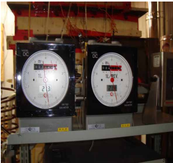
Picture 11: Dry gas meter
