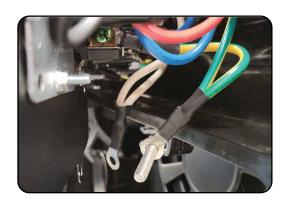
**TO THE INSTALLER:** If connecting the generator to a standard 2-pole transfer switch or interlock, then it would be advised to remove the generator bond before making the connection.
