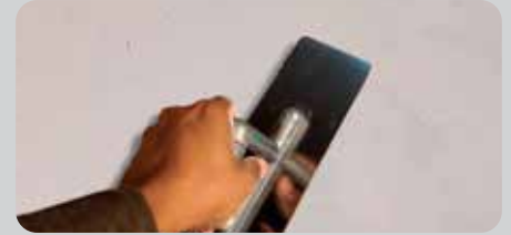
APPLY INTERIOR FILLER (3 Coats), Sand the wall and dust it off
