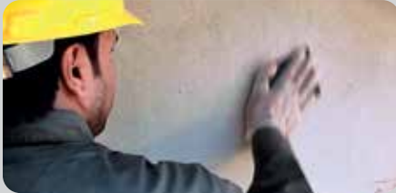
SAND THE WALL with Stone and Sand Paper Dust it off
