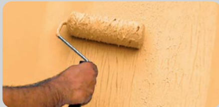
APPLY BASE COAT Brighto Super Mastic Matt
