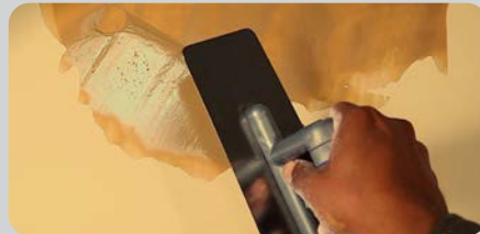
APPLY BRIGHTO PERLATA with steel trowel (3 Coats)
