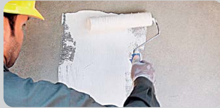
APPLY INTERIOR PRIMER with roller and allow it to dry
