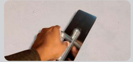
APPLY INTERIOR FILLER (3 Coats), sand the wall and dust it off
