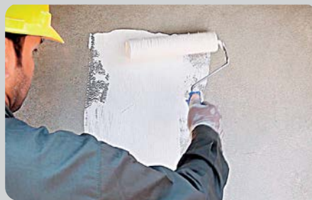
APPLY INTERIOR PRIMER With roller and allow it to dry
