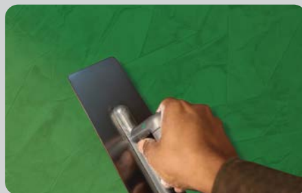
APPLICATION of Steel Trowel Cornish
