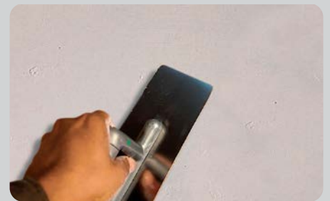
APPLY INTERIOR FILLER (3 Coats), Sand the wall and dust it off
