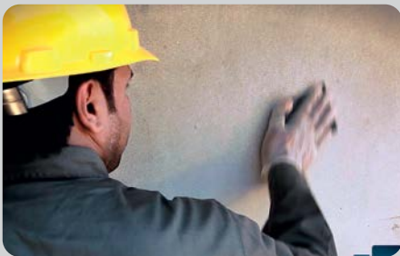
SAND THE WALL with Stone and Sand Paper Dust it off
