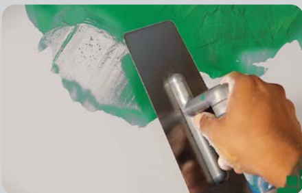
APPLY ANTIQUA POLISH PLASTER with Steel Trowel (3 Coats)
