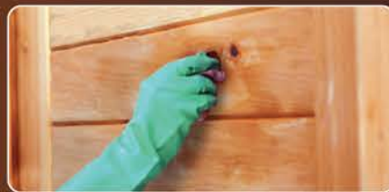
APPLY BASE COAT of All Wood Coat Sealer
