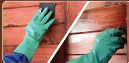
SCUFF WITH USED SAND PAPER dust it off, Apply 2 nd & 3 rd coat of AWC
