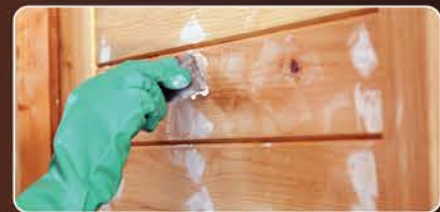
SPOT FILLING with the help of spatula
