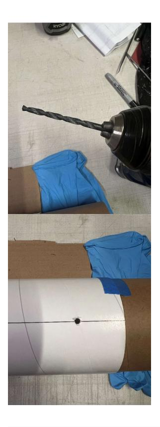
Now I remove the tape and pull the coupler out of the tube. At this point I put some CA around the holes I drilled. See pictures. Let this harden up and the sand the burrs off.
