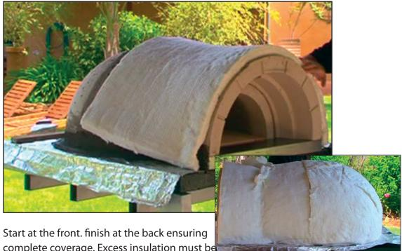
complete coverage. Excess insulation must be used to plug gaps. Cut a hole for the flue.
