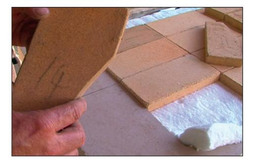
Measure back from front floor piece 655mm . Mark foil both sides of slab.
