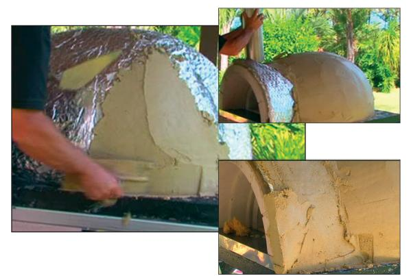
**Insert the flue into the front chamber hole with the seam of the flue facing the back of the oven before beginning the rendering process.** Use a spirit level to ensure the flue remains straight. For best results. use a steel float to apply the render mix. What can go wrong?
