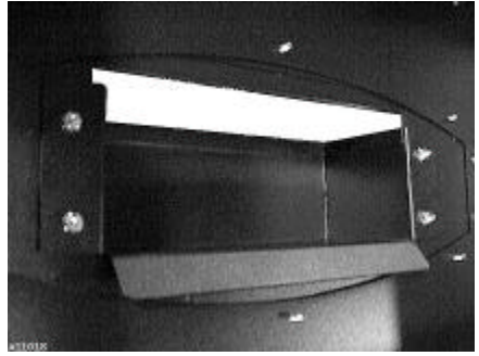
Figure 17. Install and tighten nuts.
