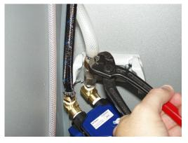
9) Push both sections of tubing onto the barbed fittings and pinch the hose clamps to seal/secure
