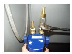
7) Install the 2 x 3/8" fittings into the Purity C head, noting the double non-return valve fits to the inlet port (see direction arrows on top surface of molding)
