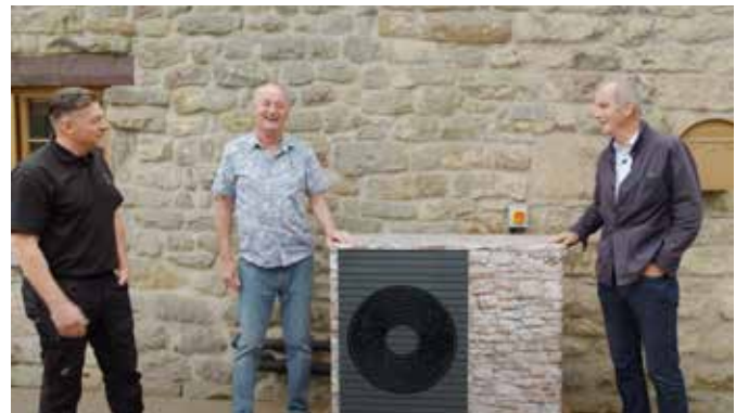
Heat Pump Possible : South Barn
