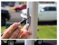
STEP ONE: Position the Cleat(s) 3-4ft from the bottom of the flagpole. Or to your preferred height. With a pencil or marker, mark where the holes will be.
