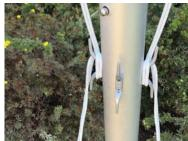
Once your yardarm is installed on your flagpole, tie the loose ropes to the cleats that you previously installed.
