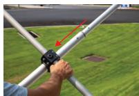
STEP FOUR: Extend the 1st and 2nd top sections of the pole. Slide the yard arm onto the pole and align with the previously drilled hole.
