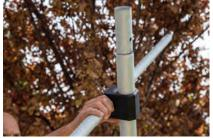
STEP THREE: Slide the yard arm onto the pole and align with the previously drilled hole.
