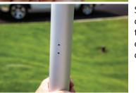
STEP TWO: Use a 9/64" drill bit to drill holes into the marked locations. Use extreme caution when drilling into your flagpole.
