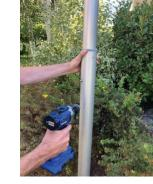
STEP EIGHT: Use a 9/64" drill bit to drill holes into the marked locations.
