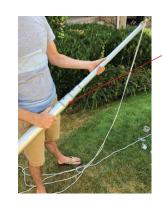
STEP SIX: Extend the first (bottom) section of the flagpole. (this is important so you don't drill through multiple sections)
