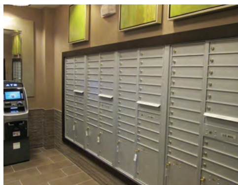
Apartment Community - Washington DC
