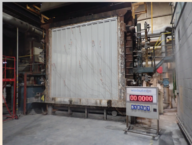
FIREWALL AT START OF TEST
