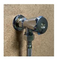
Step 1- Identify the cold water tap which feeds the washing machine. Turn stop tap clockwise to turn the water off to the washing machine. Un-thread the attached water line feeding to the washing machine.
