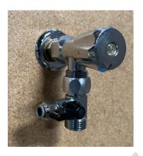
Step 2- Pictured is the washing machine ¾" adapter installed onto the washing machine stop tap. Please note the supplied washer needs to be installed in the Female thread of the adapter (Between stop tap and adaptor). Adaptor only needs to be done up finger tight and generally ¼ turn with a spanner is all the is required to make the correct seal. Please note some adaptors will have a chrome ball valve handle. No thread tape is required with any of the fittings/connections.
